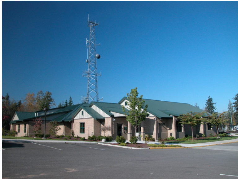
Valley Communications Center Kent, Washington
